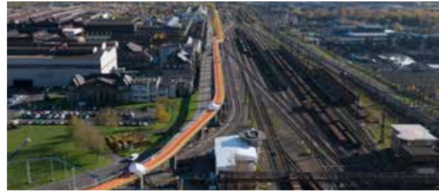
The new bridge winds between our Belval site and the railway line. Three areas of expertise at ArcelorMittal, from beams to double-curvature T-sections
