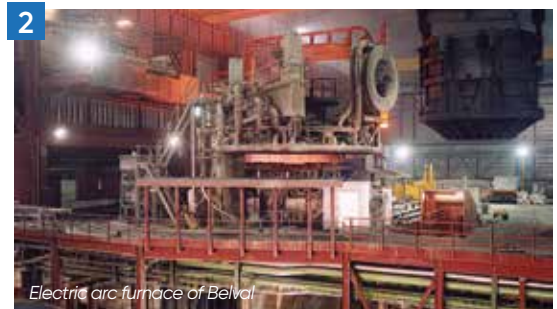
Electric arc furnace of Belval
